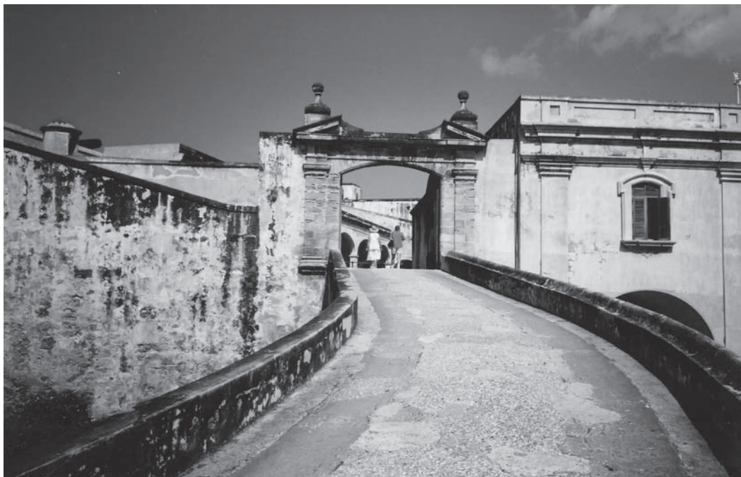
Fig. 2. Main entrance to the fort through the North Gate
