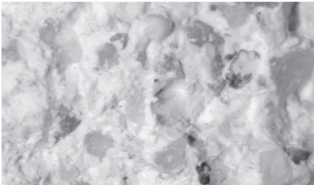
Fig. 11. Interior surface of mortar sample 14M200 under low magnification. The binder is very white, which is aesthetically consistent with a render that is meant to be seen.
